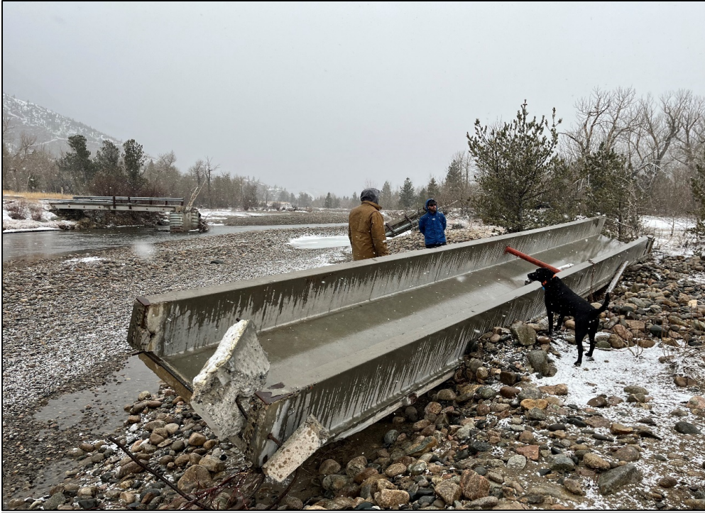
Figure 85. View upstream of failed bridge debris lodged on channel margin, Rainbow Subdivision bridge, upper Stillwater River.
