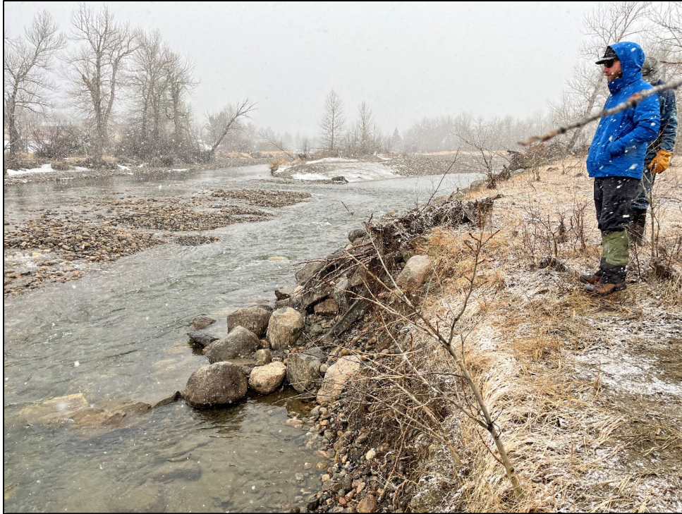
Figure 68. View upstream of local erosion on end of riprap; local use of wood can effectively deflect flows from bankline of concern and provide habitat.
