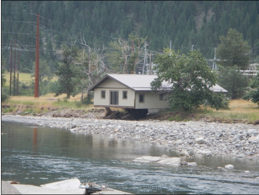
Figure 56. Undermined structure on Stillwater River upstream of Nye as viewed in late August 2022.
