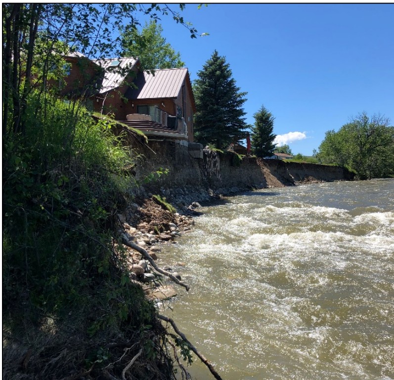
Figure 72. High bank residence being actively undermined during flood, Stillwater River.
