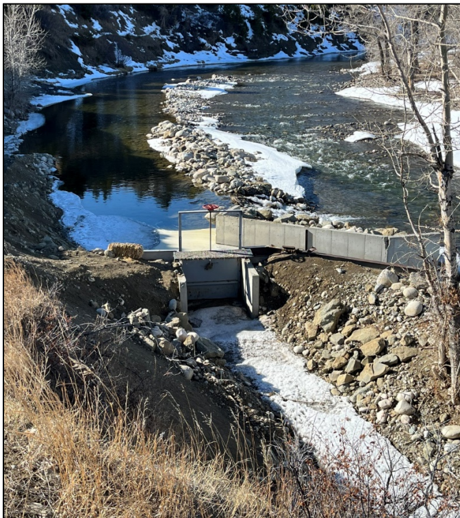
Figure 88. View upstream of Yanzik Diversion that experienced major abutment erosion during flood.
