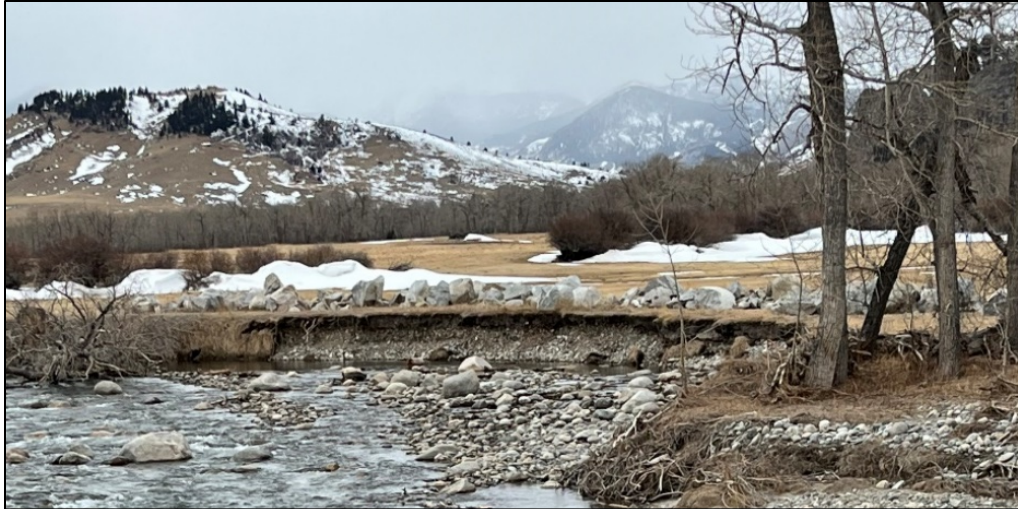
Figure 66. Large riprap staged on bankline; note lack of infrastructure threat and relatively passive bank margin post-flood.
