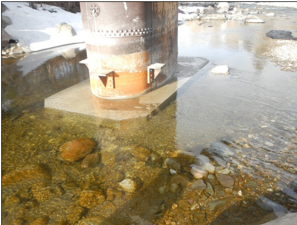
Figure 84. Bridge pier above Cliff Swallow FAS replacing one that was undermined during flood event, causing bridge to deck to buckle but not fail.
