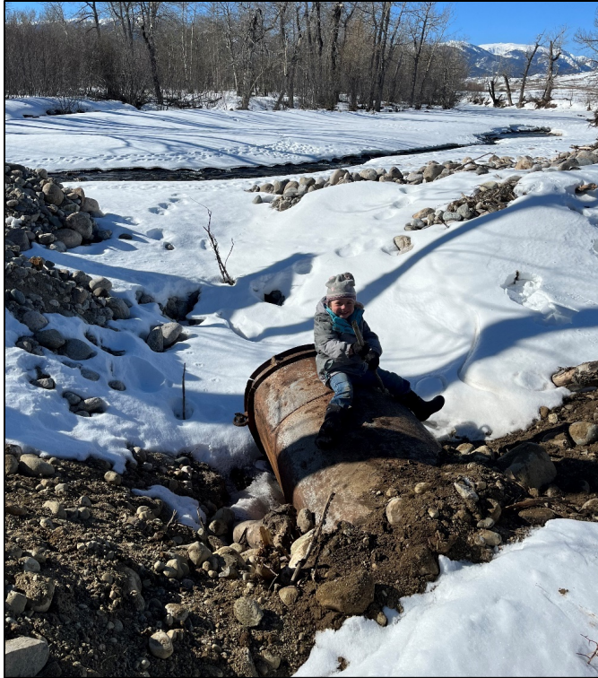
Figure 89. Diversion intake that experienced erosion damage; the bank was rebuilt with a cobble berm.
