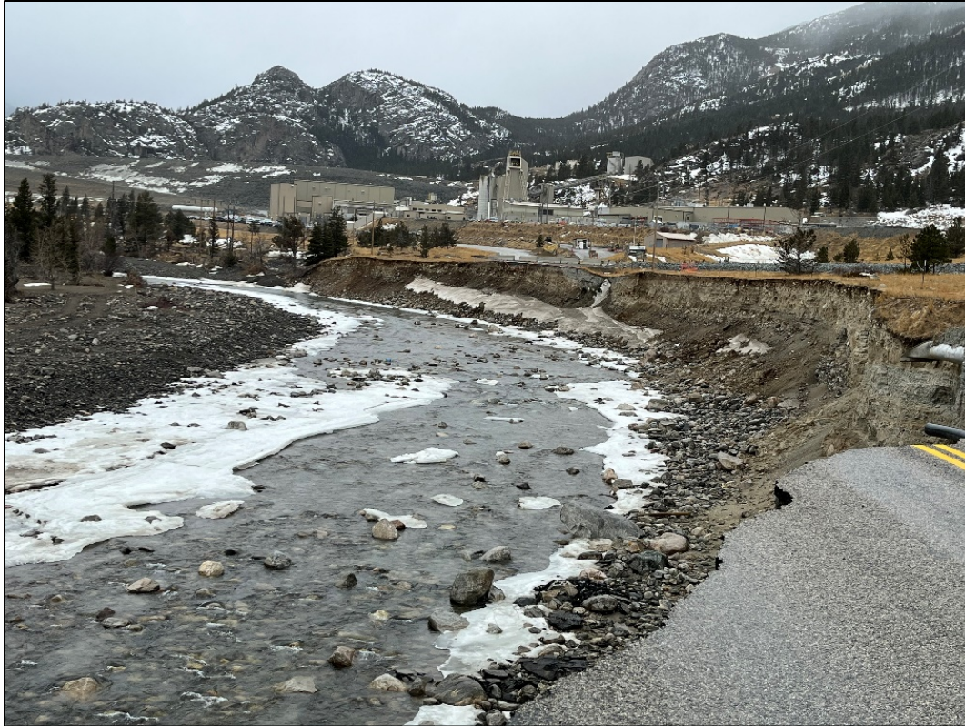
Figure 57. Road damage on upper Stillwater River near the Sibanye-Stillwater Mine (March 2023).
