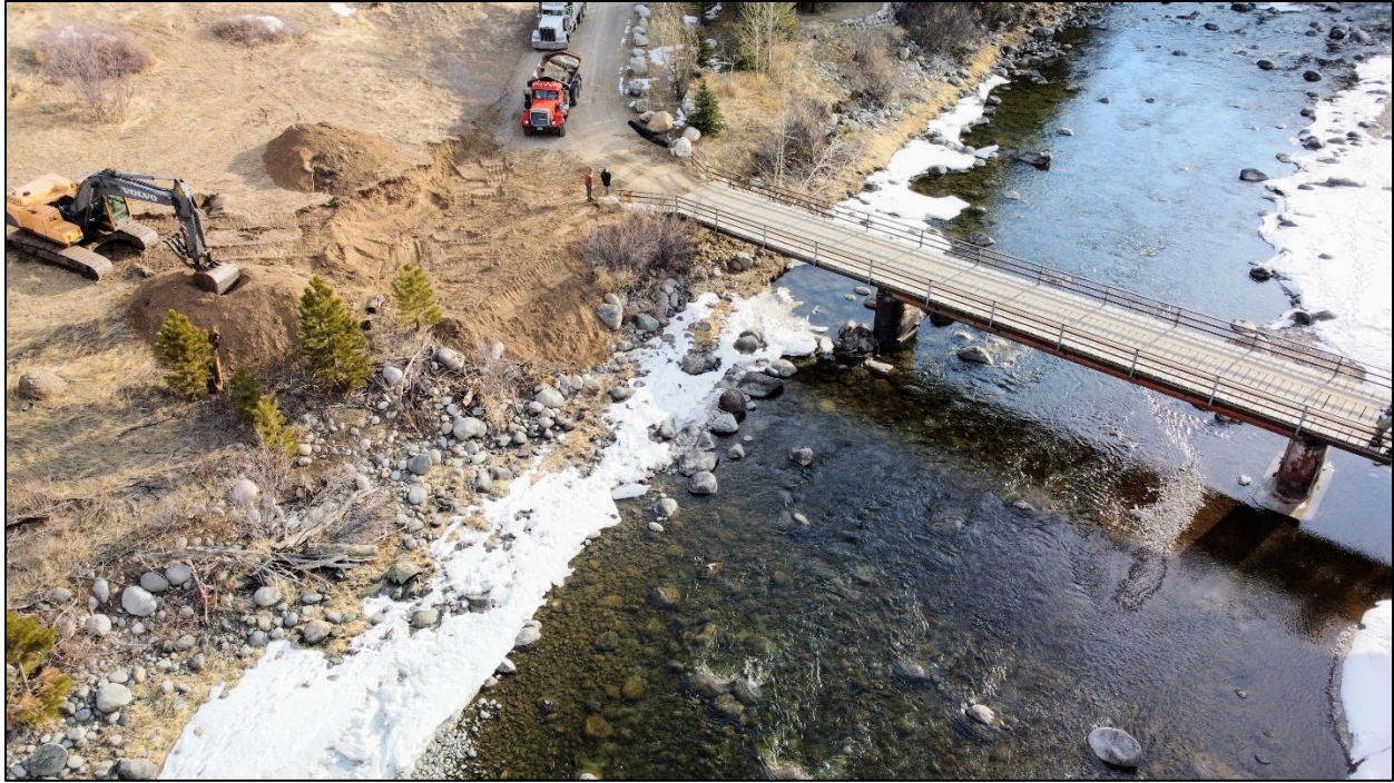
Figure 83. Active bridge abutment riprap reinforcement, Stillwater River.
