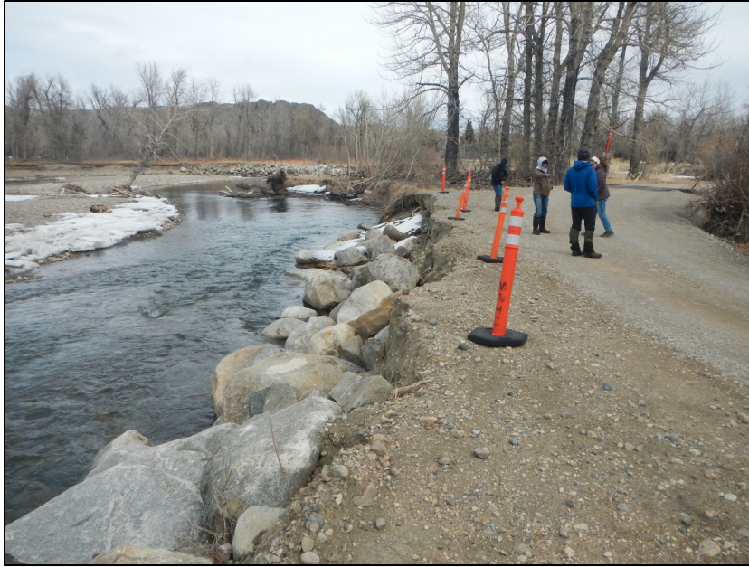
Figure 80. Flood damaged gravel access road margin on upper Stillwater River; this rock is on an over-steepened bank which will need to be regraded to remain stable.
