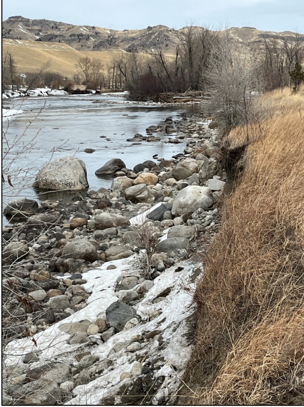
Figure 74. Coarse native boulder toe accumulations provide natural armor, no action recommended.
