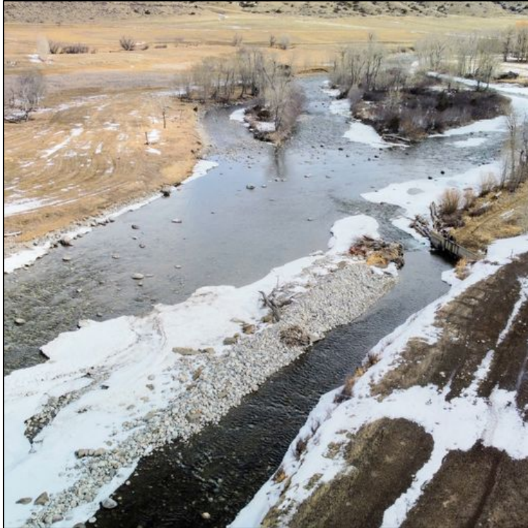
Figure 87. View downstream showing Mendenhall Ditch Co. diversion that experienced major debris/sediment accumulations at headgate; material has been removed and structure is slated for additional repairs.
