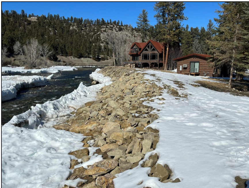
Figure 67. View downstream on lower Stillwater showing recently armored bankline extending above natural floodplain elevation.
