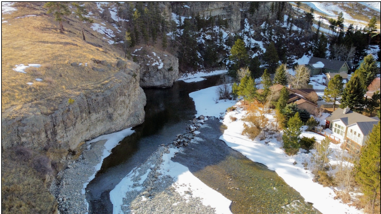
Figure 90. View upstream of rock diversion on the Stillwater River above Cliff Swallow spanning the entire channel. This diversion channel could be narrowed and extended upstream closer to the bedrock bank which would maintain flow and bedload transport capacity in the main channel.
