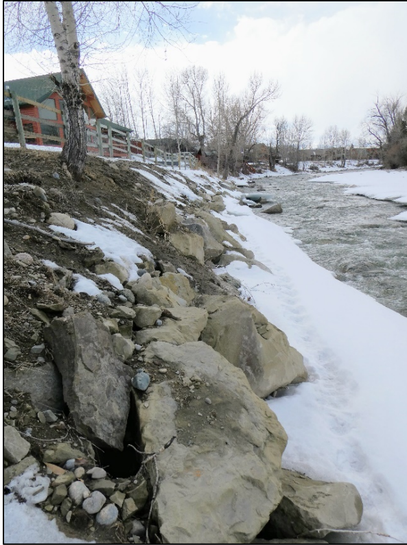
Figure 76. Steep bankline that was repaired under emergency status due to threat to property. This type of project can deteriorate and may not survive subsequent runoff events.
