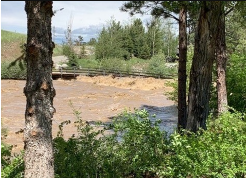
Figure 82. Private bridge along the Stillwater Road overtopping during flood (courtesy of Staci Grimm).
