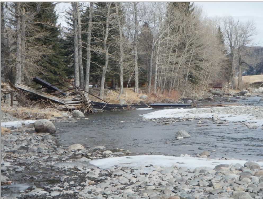
Figure 86. Small access bridge debris within active channel, middle Stillwater River.
