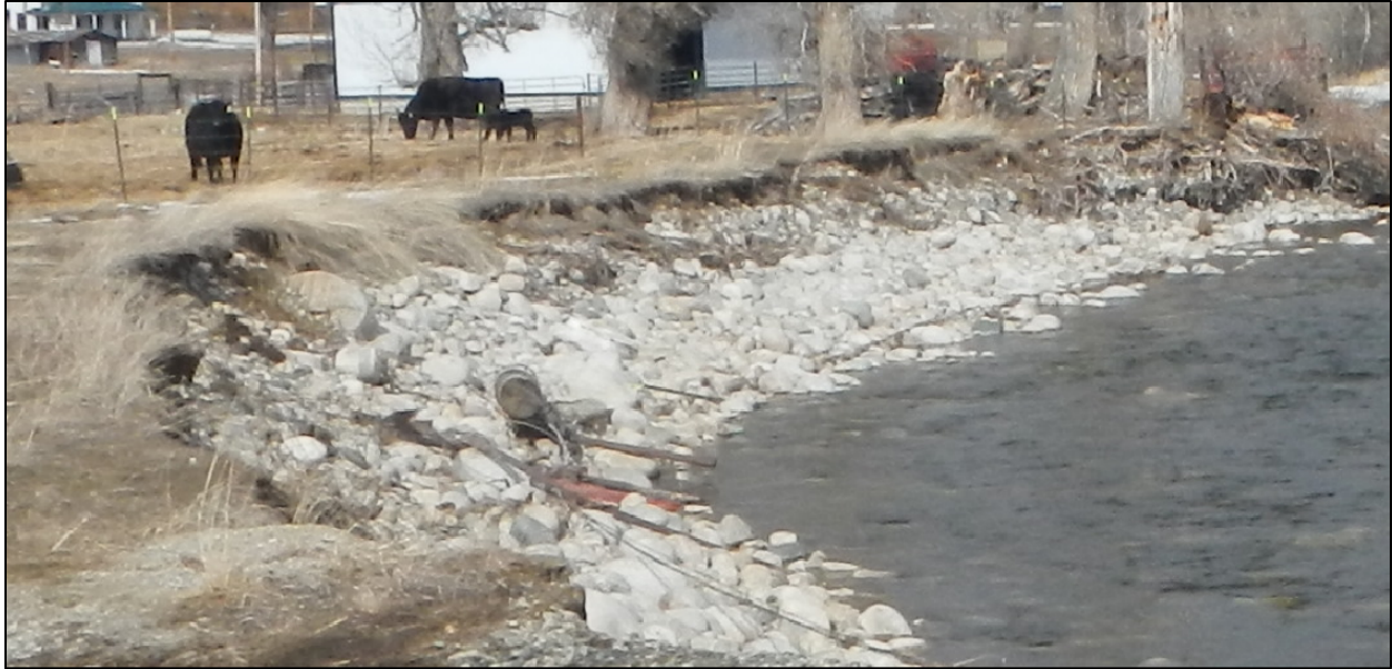
Figure 70. Natural analog for using locally derived rounded boulders to reinforce bank toes.
